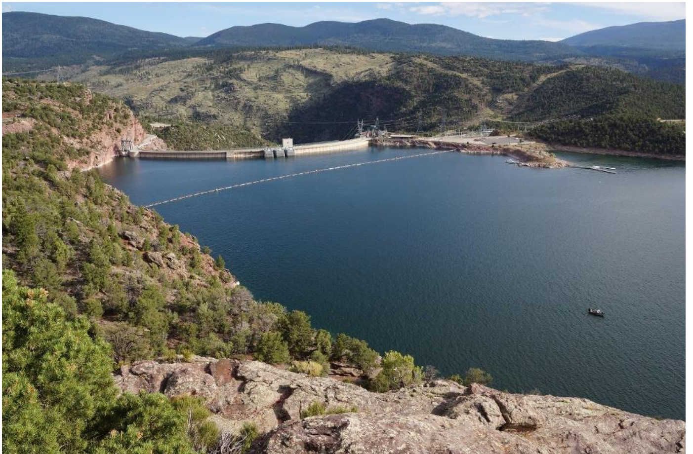
The 502' by 1,285' foot Flaming Gorge Reservoir Dam.
