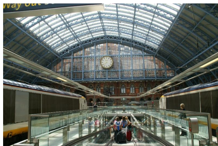
Above: The Paris train station for taking the “Chunnel Train” to London. Right: The London train station destination.
